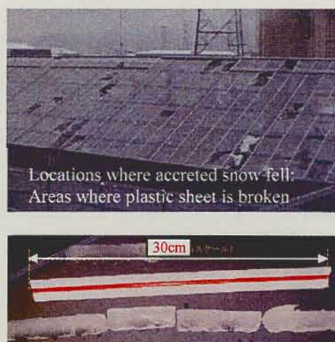
Fig. 1. An example of Damage to a greenhouse from fallen accreted snow
